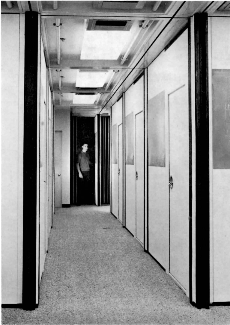
FIGURE 2. THE EXPERIMENTAL AREA PARTITIONED INTO 7' \times 7' EXPERIMENTAL CUBICLES. SOUND-BAFFLED AIR CONDITIONING OUTLETS, T.V. MOUNTING RACKS, AND TRACKS FOR THE PANELS ARE VISIBLE IN THE CEILING.
